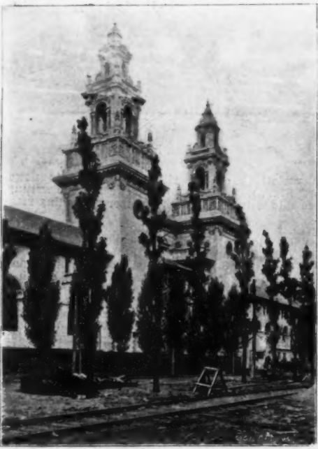
NORTHERN FAÇADE, MACHINERY BUILDING.
